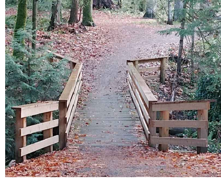
COLLIERY DAM FENCE INSPIRATION
